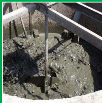
Biogas and Anaerobic Reactors
